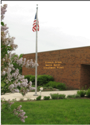
French Creek Waste Water Treatment Plant North Ridgeville, OH
